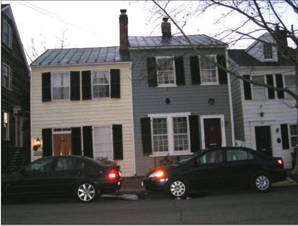
Figure 1. Front (east) elevation of 607 South Fairfax Street (left).
