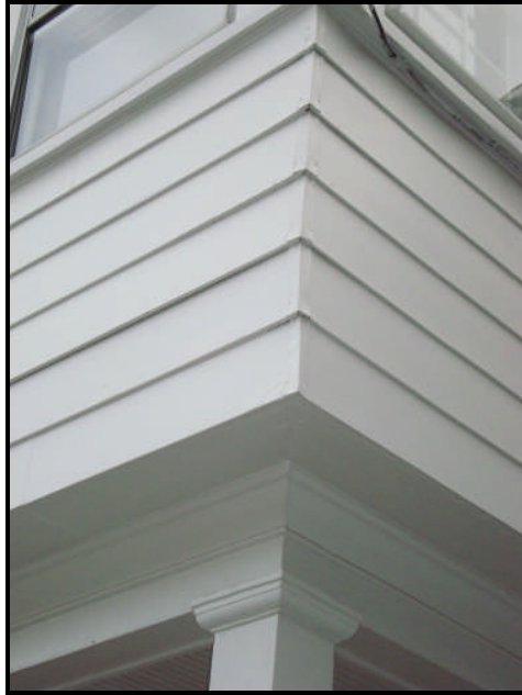
Figure 16. Rear Second-Story Addition's Cement-Fiber Siding
