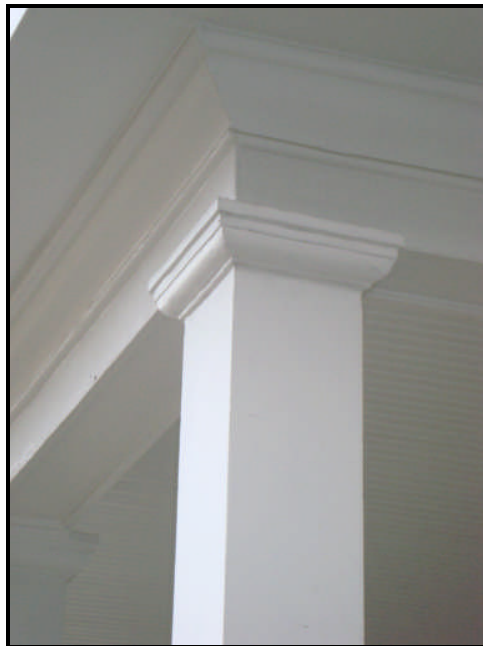
Figure 17. Rear Second-Story Addition's Column Detail
