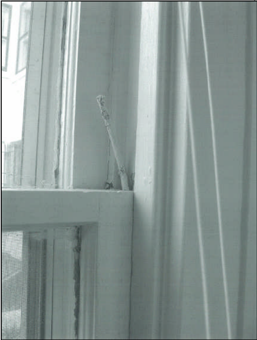
Figure 6. Window Survey: Existing Conditions-Interior of Main Massing
