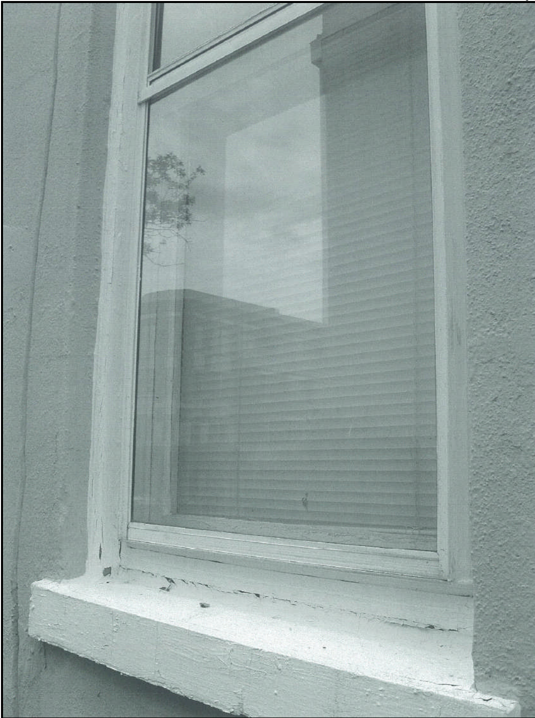
Figure 3. Window Survey: Existing Conditions-Exterior of Main Massing
