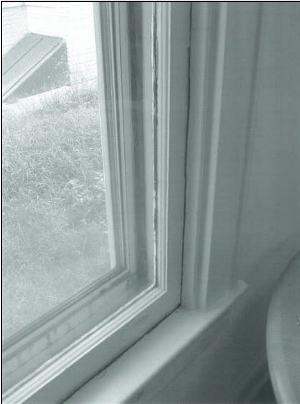
Figure 8. Window Survey: Existing Conditions-Interior of Frame Addition
