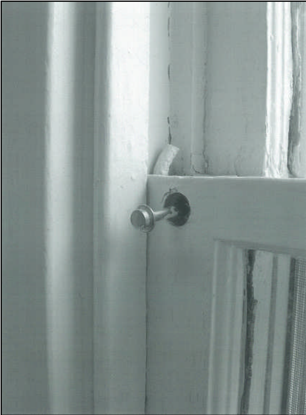
Figure 5. Window Survey: Existing Conditions-Interior of Main Massing
