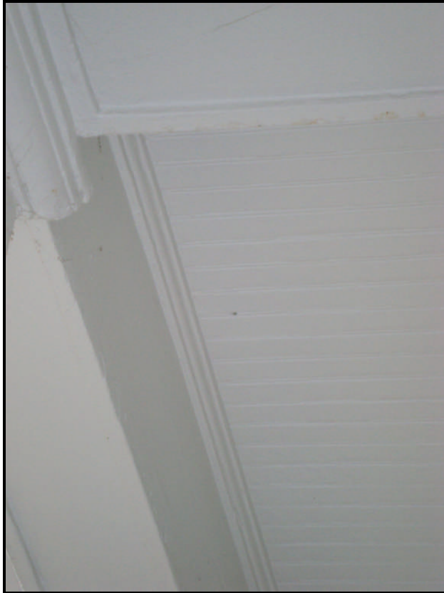
Figure 18. Rear Second-Story Addition's Ceiling
