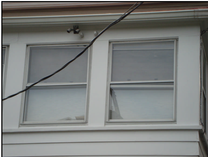
Figure 15. Rear Second-Story Addition's Windows
