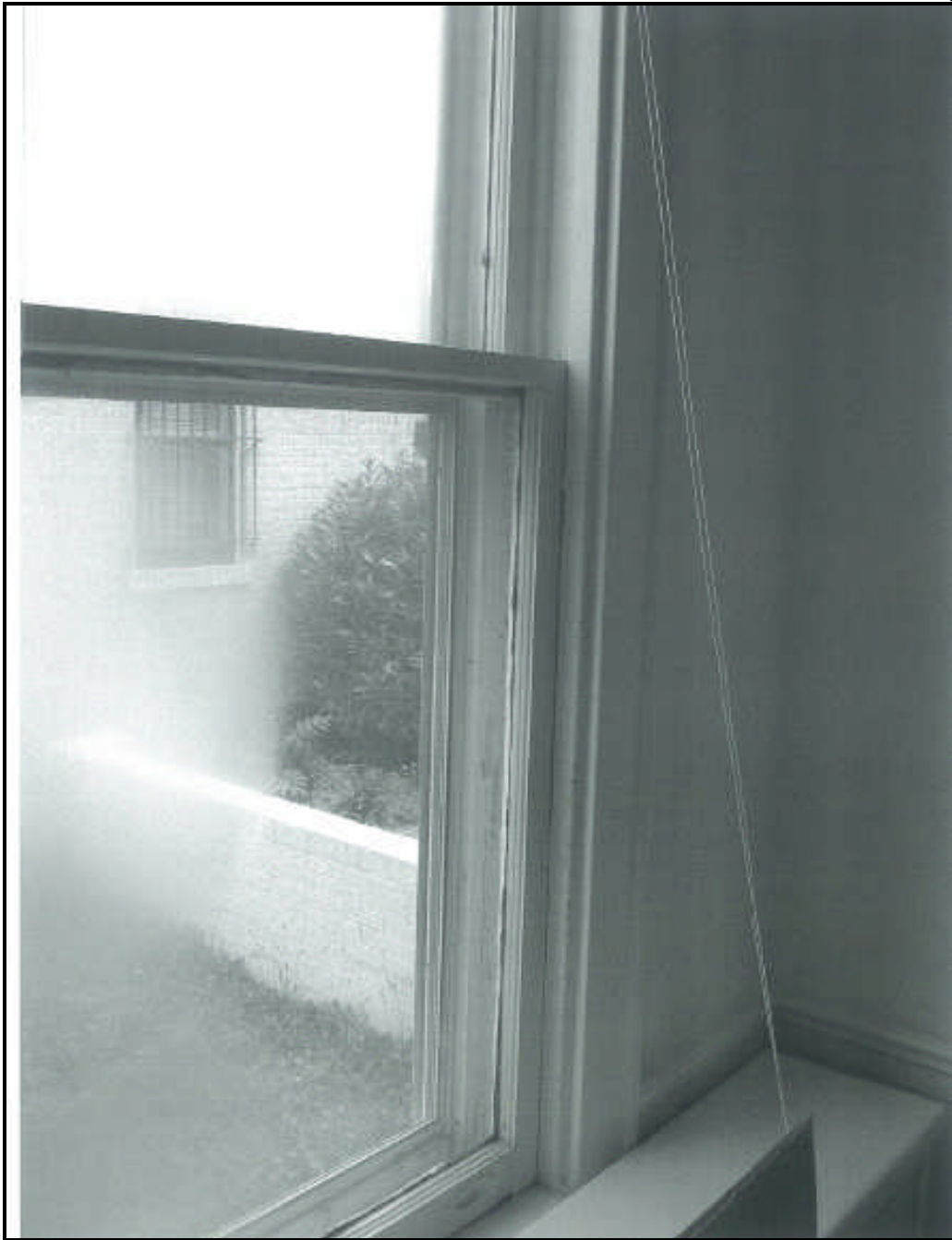
Figure 7. Window Survey: Existing Conditions-Interior of Frame Addition
