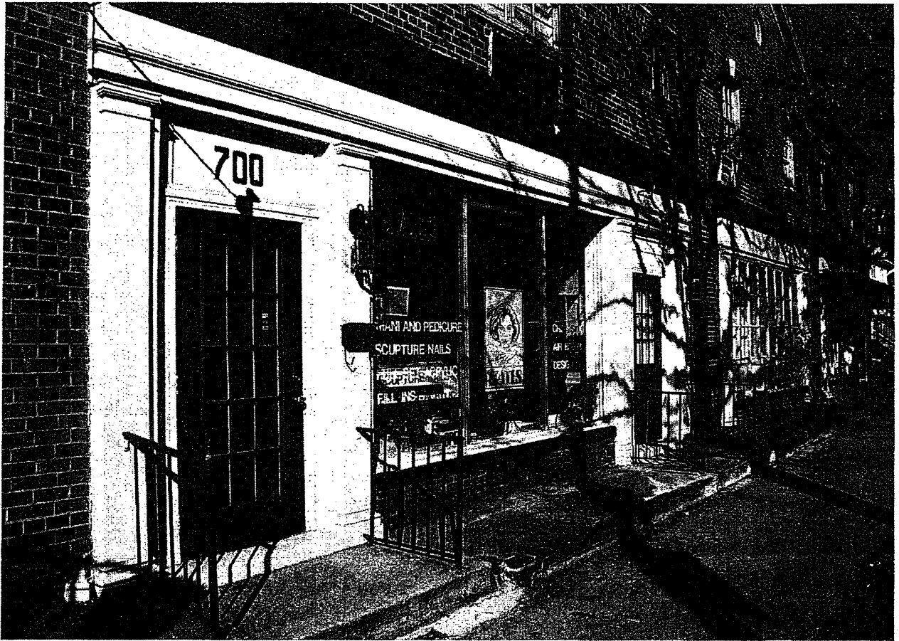
Exhibit 3a North Washington Street façade Note remnant of original cham- fered corner at lower left of picture.
