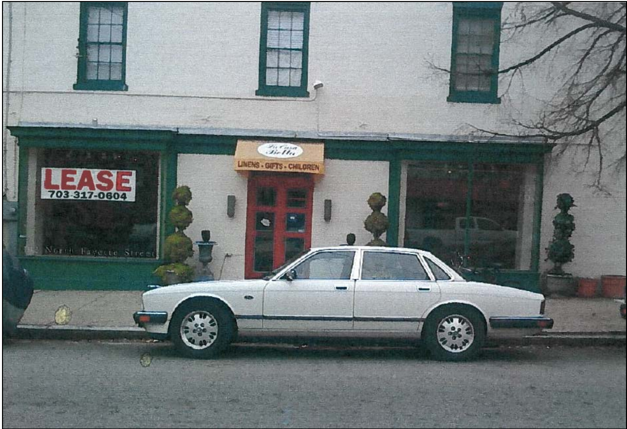
Figure 1. Existing conditions, 102 North Fayette Street.
