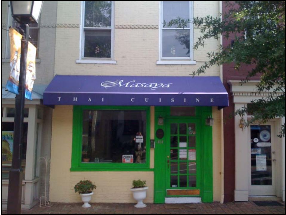
Figure 2: Photo of Existing Condition
