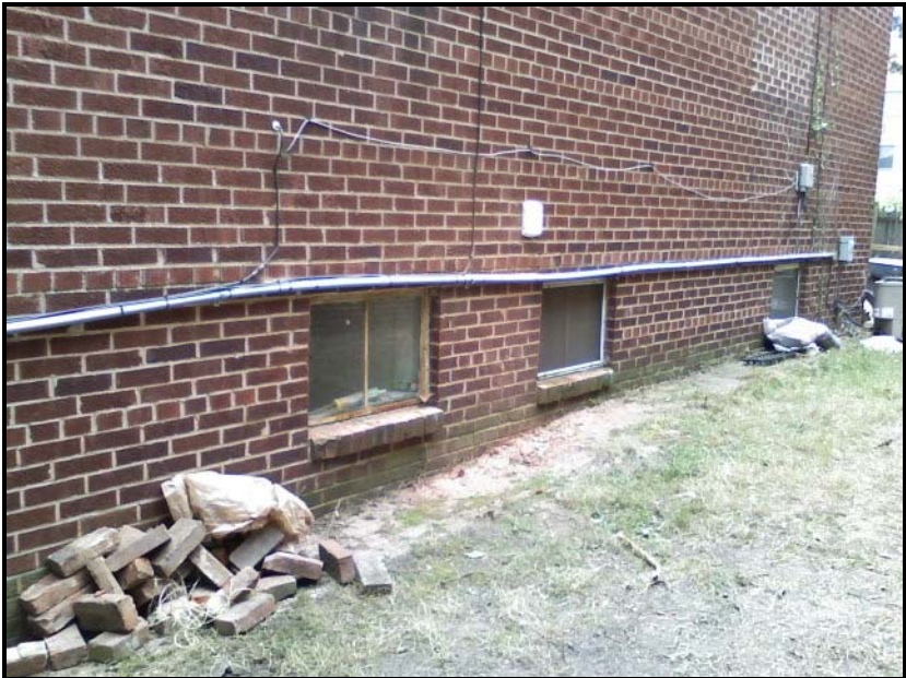
Figure 5. Photograph of basement windows on north elevation
