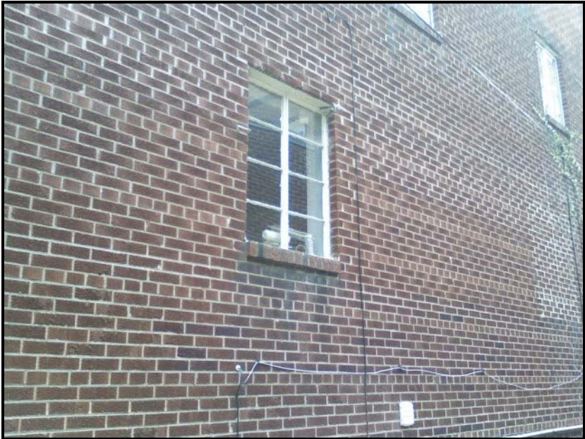
Figure 6. Photograph of casement windows on north elevation
