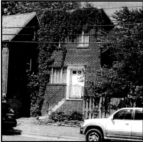
Figure 1. Photograph of front elevation
