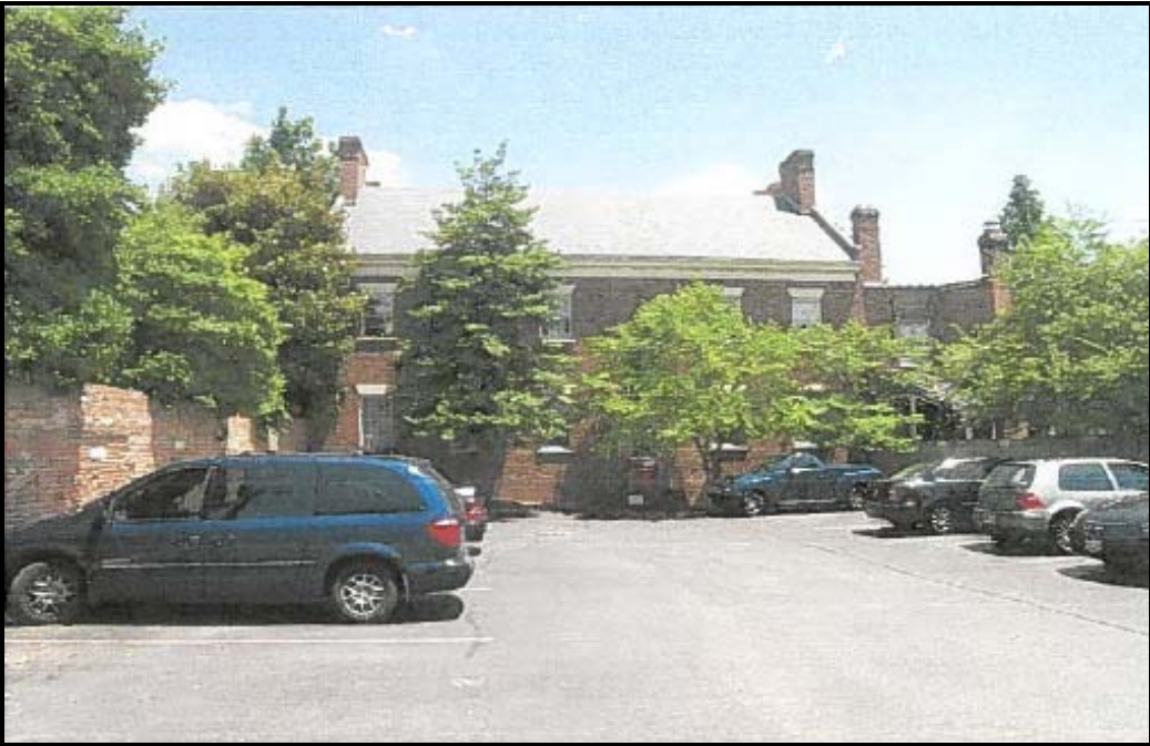
Figure 4: Photo of Existing Rear Facade
