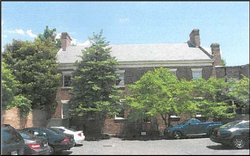
Figure 3: Photo of Existing Rear Facade
