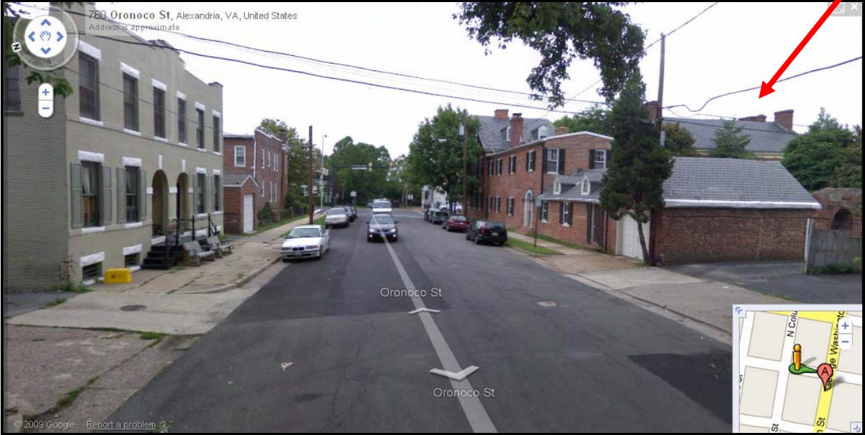
Figure 5: View from Oronoco Street - Looking at rear roof slope of 424 N. Washington Street
