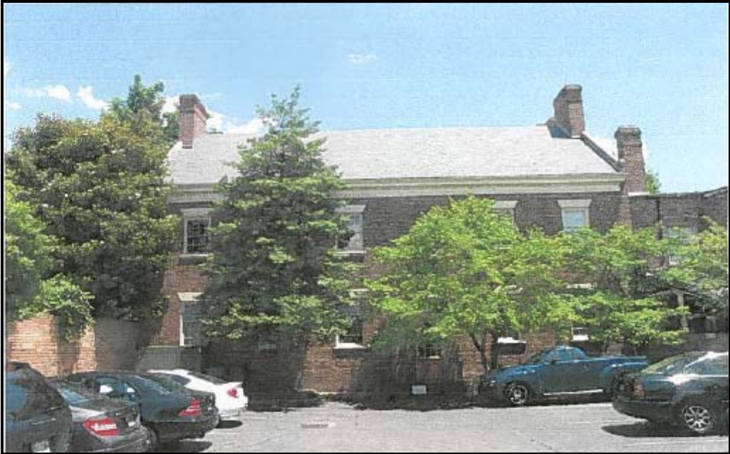
Figure 3: Photo of Existing Rear Facade
