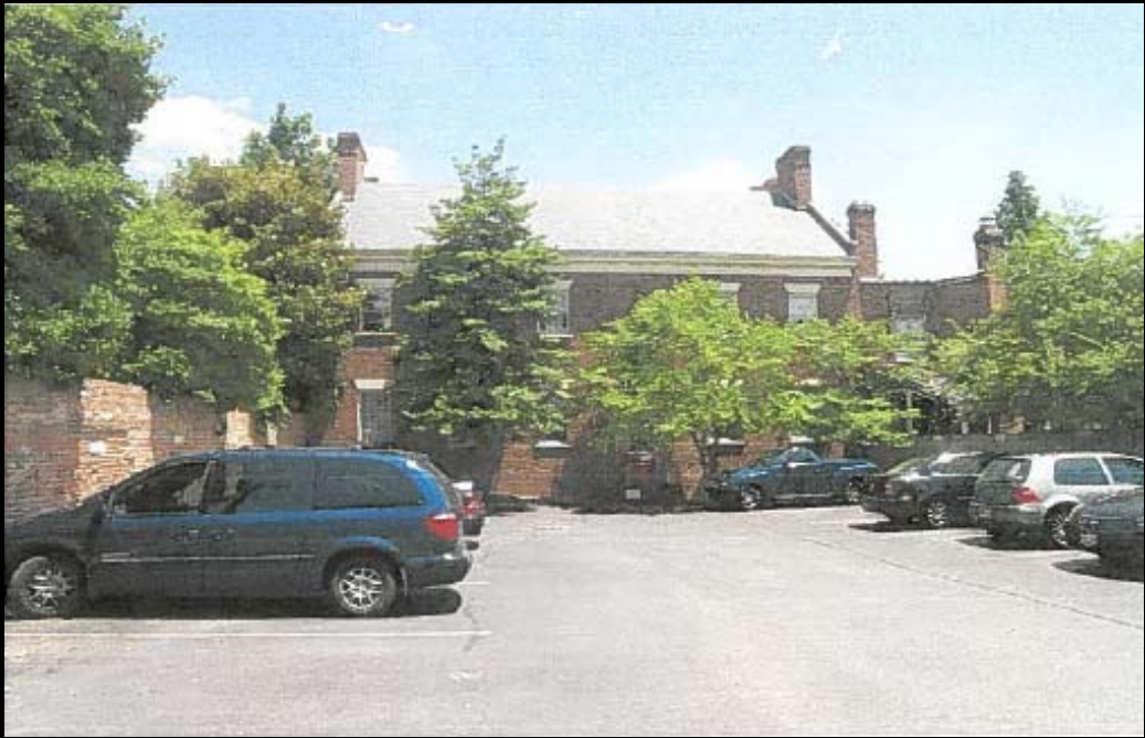
Figure 4: Photo of Existing Rear Facade
