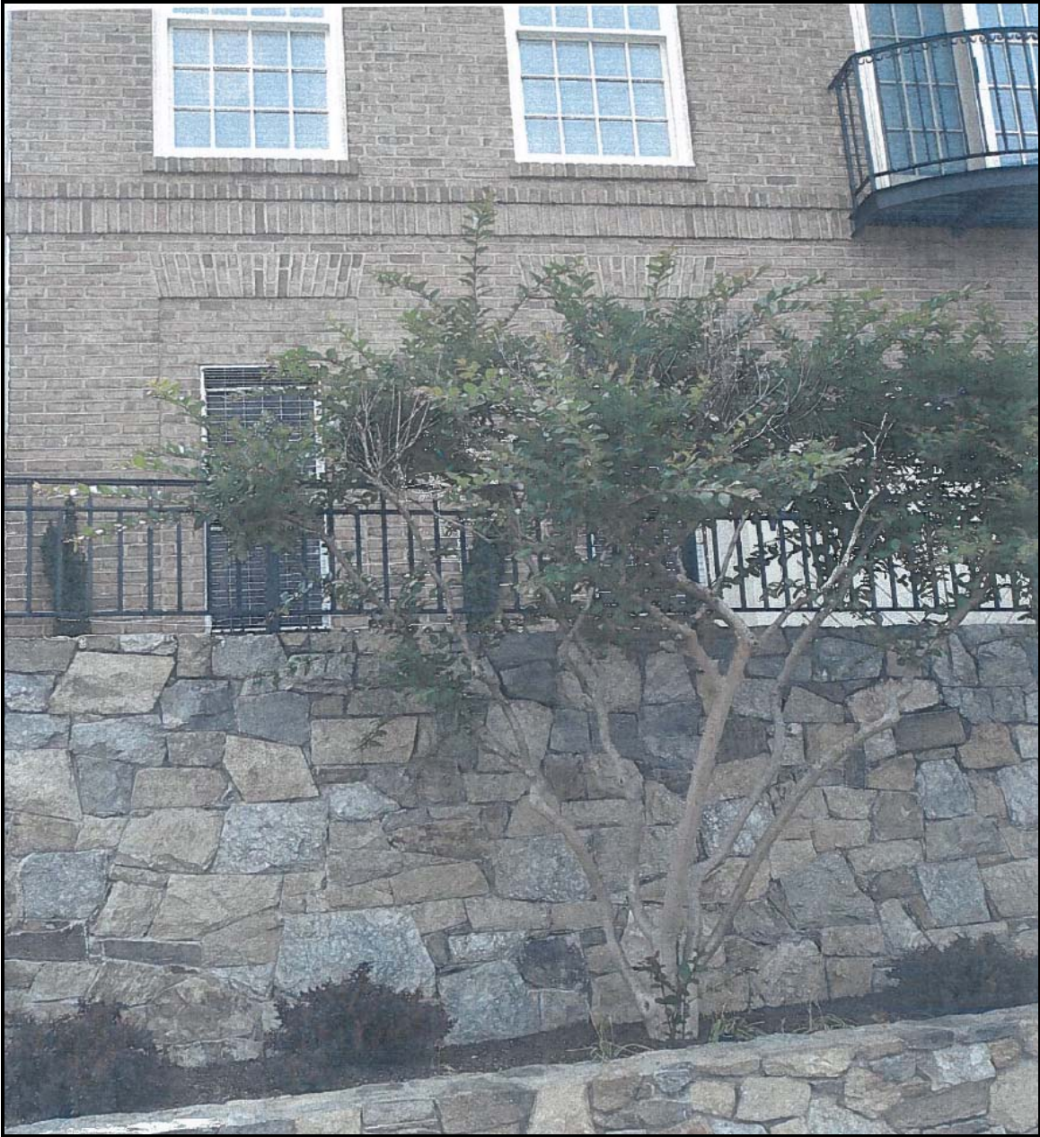
Figure 3: Photo taken from the boardwalk below showing the through-the-wall HVAC units.
