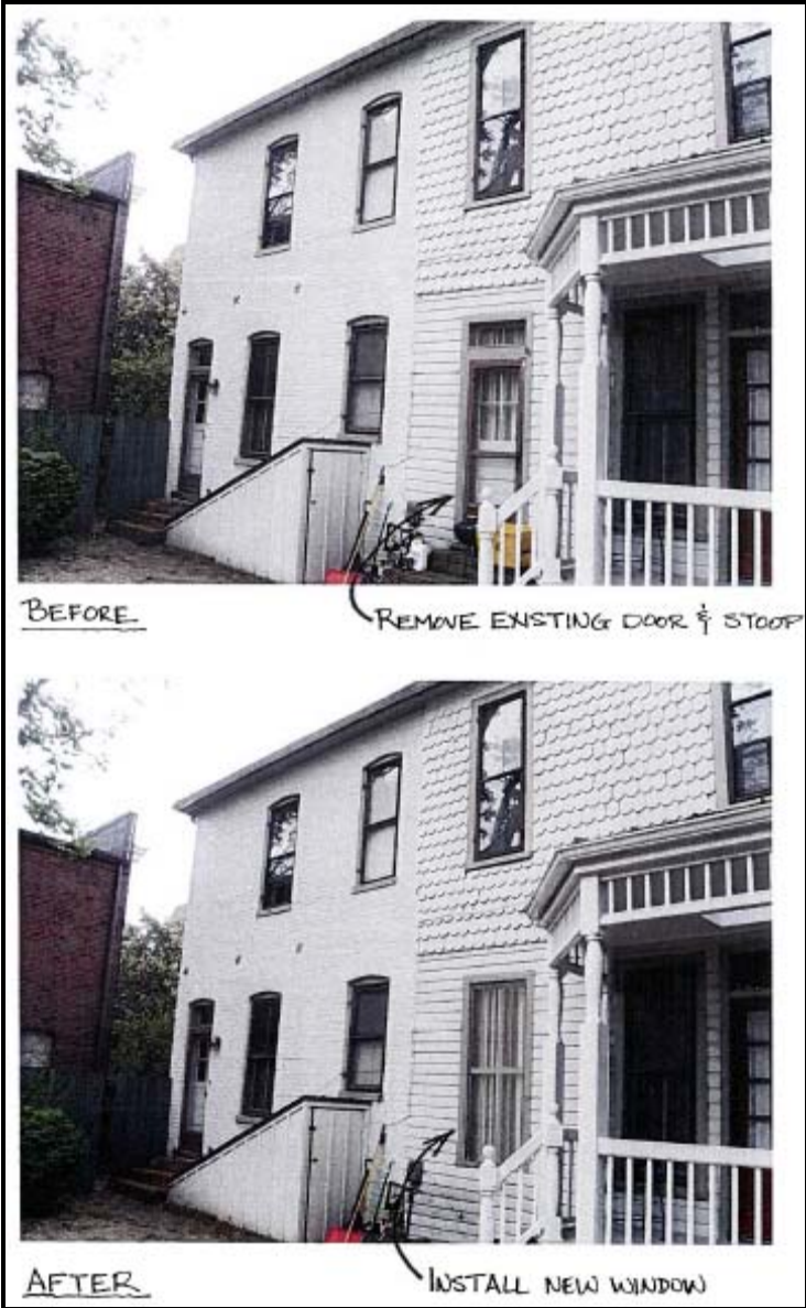
Figure 4. Photo and simulation showing proposed new window.
