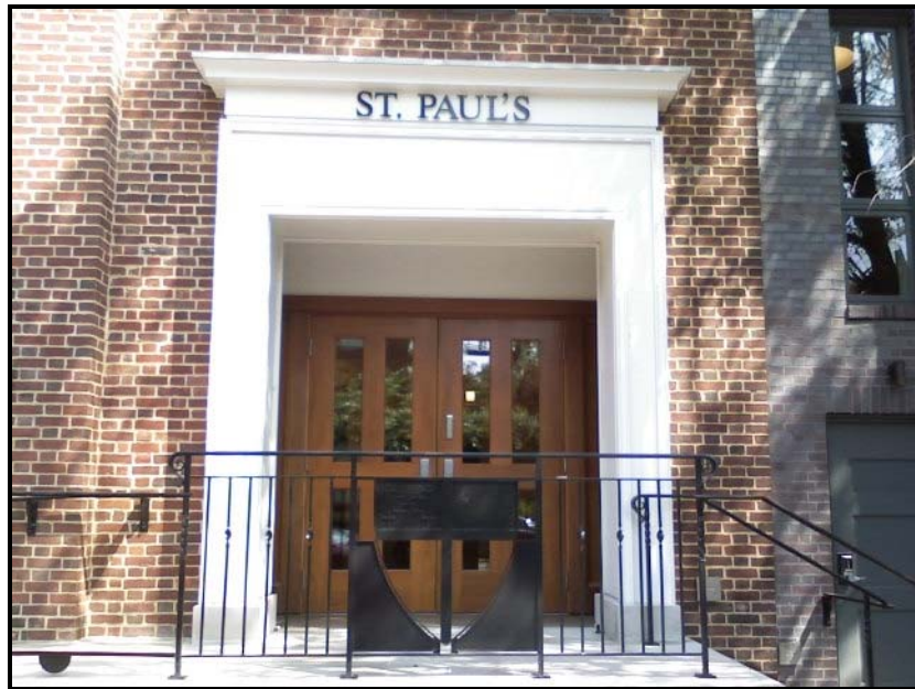
Figure 6. Photograph of Duke Street elevation.
