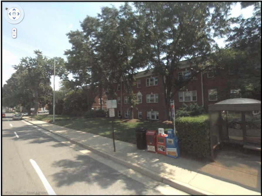
Figure 1. Photograph of building from S. Washington St.
