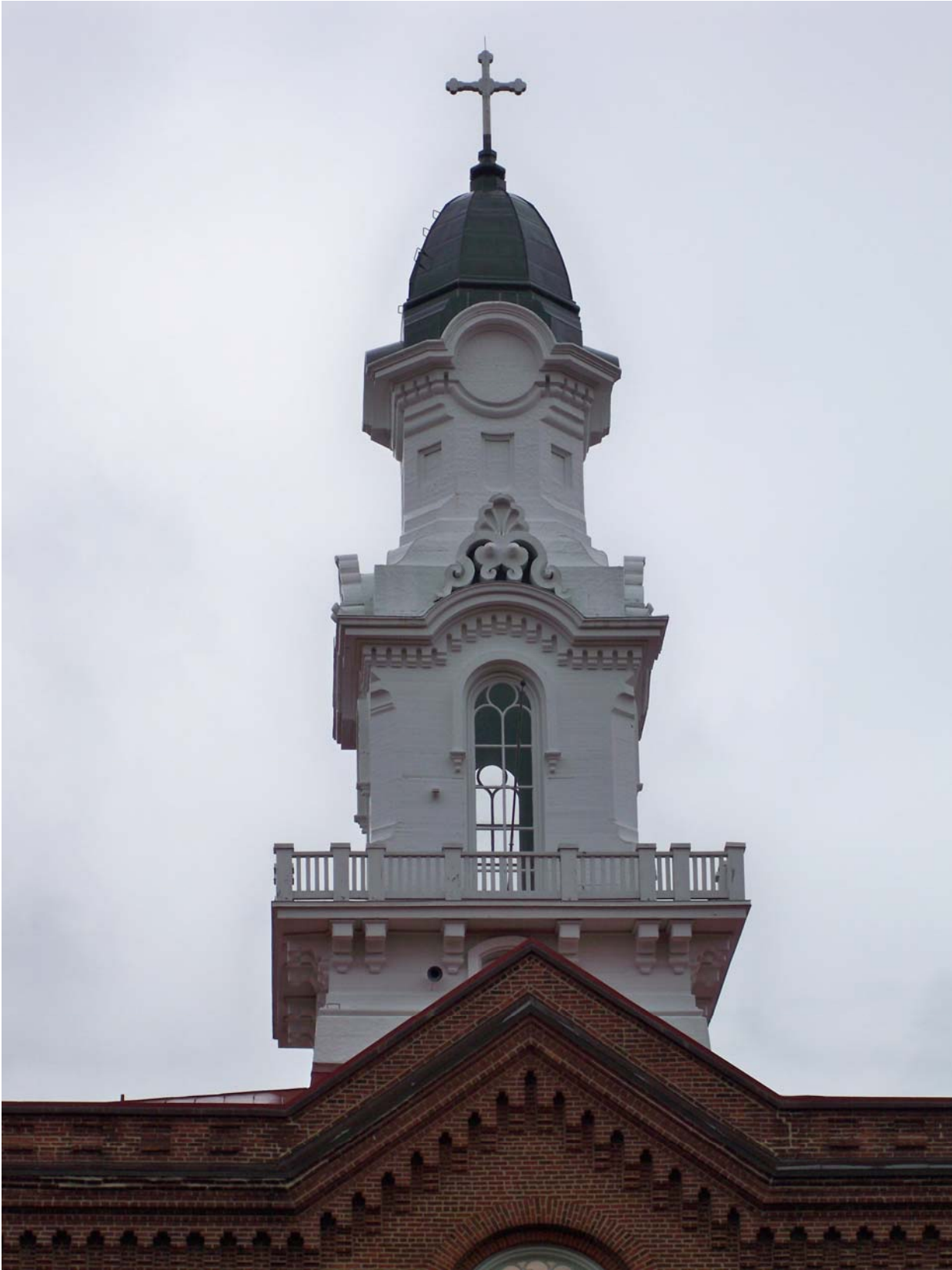
Figure 3: Existing View of Tower/Steeple
