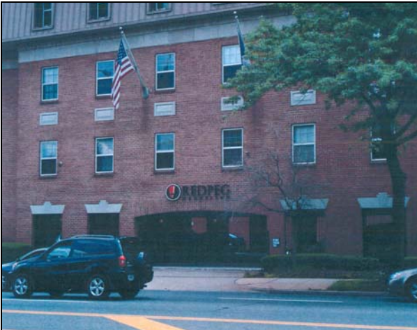
Figure 1. Existing signage on N. Washington elevation.
