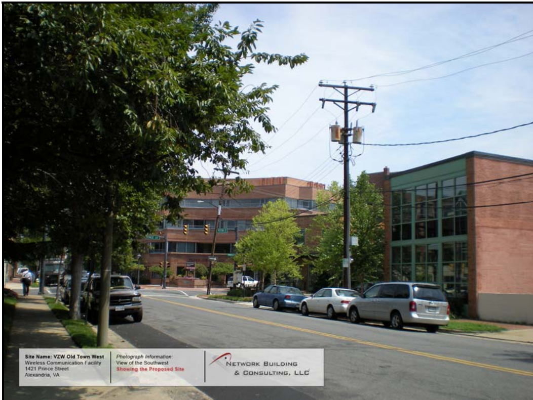
Figure 7: Existing – View of the Southwest
