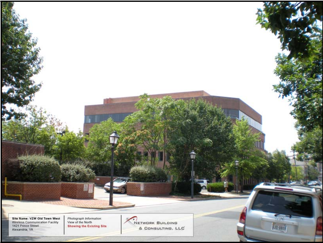
Figure 4: Existing – View of the North
