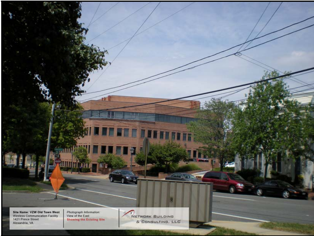
Figure 2: Existing – View of the East
