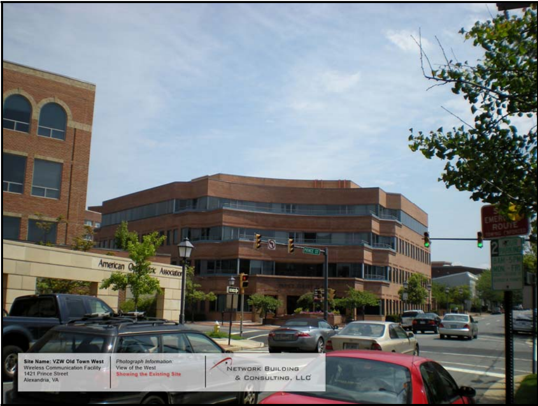
Figure 8: Existing – View from the West
