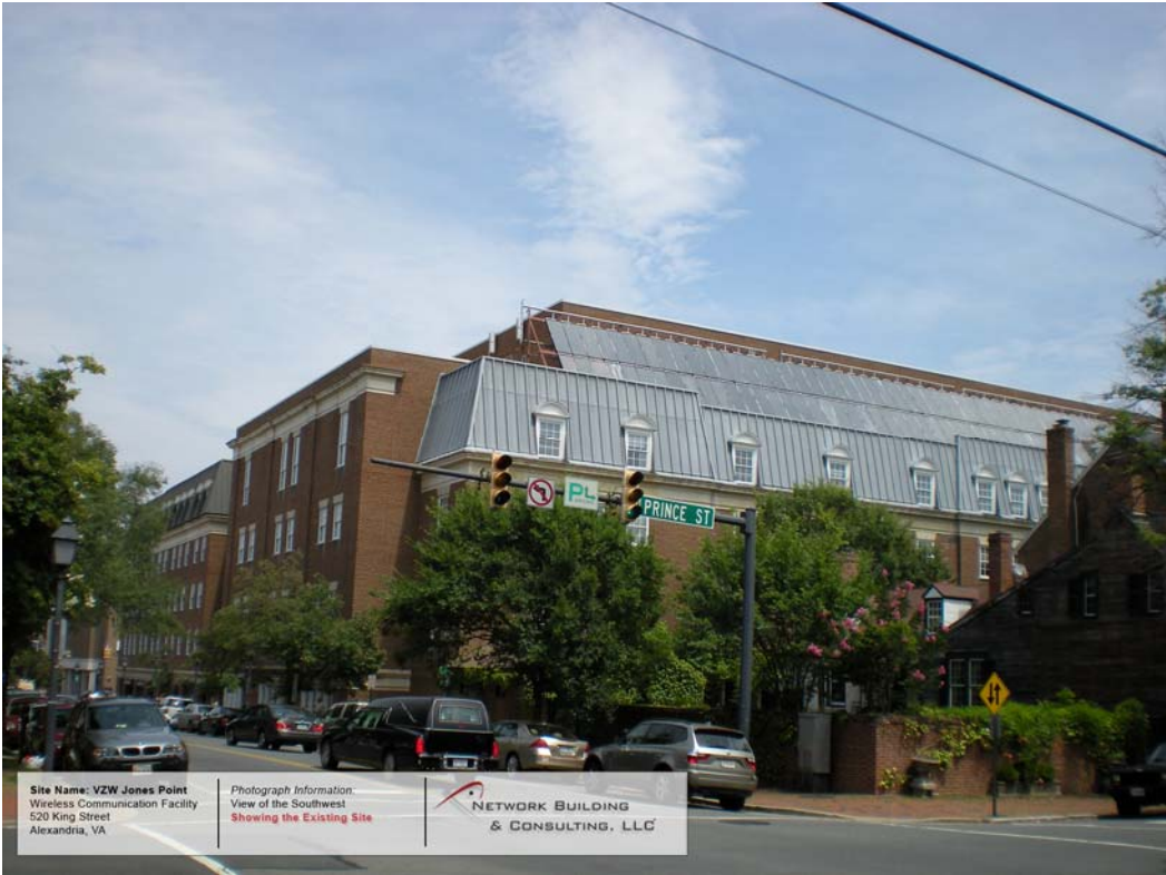
Figure 6: Existing– View of the Southwest
