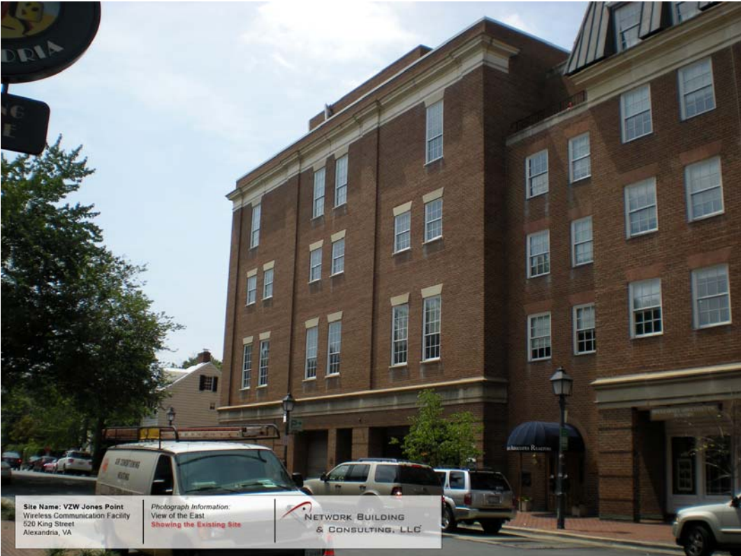
Figure 2: Existing – View of the East
