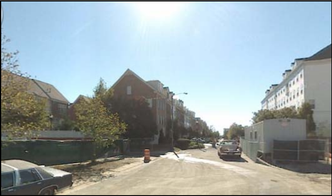
Figure 5: View of the project area
