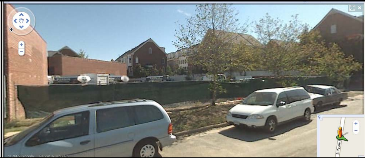
Figure 2: View of the project area
