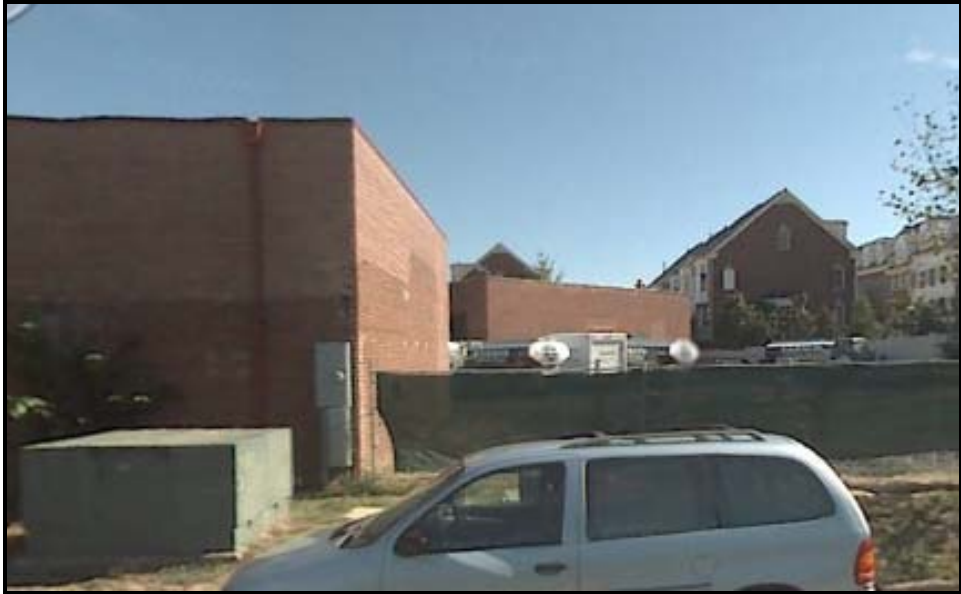
Figure 4: Views of the project area
