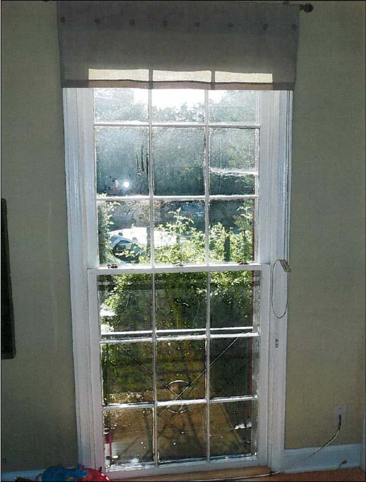
Figure 3. Interior view of window proposed for replacement on first story.
