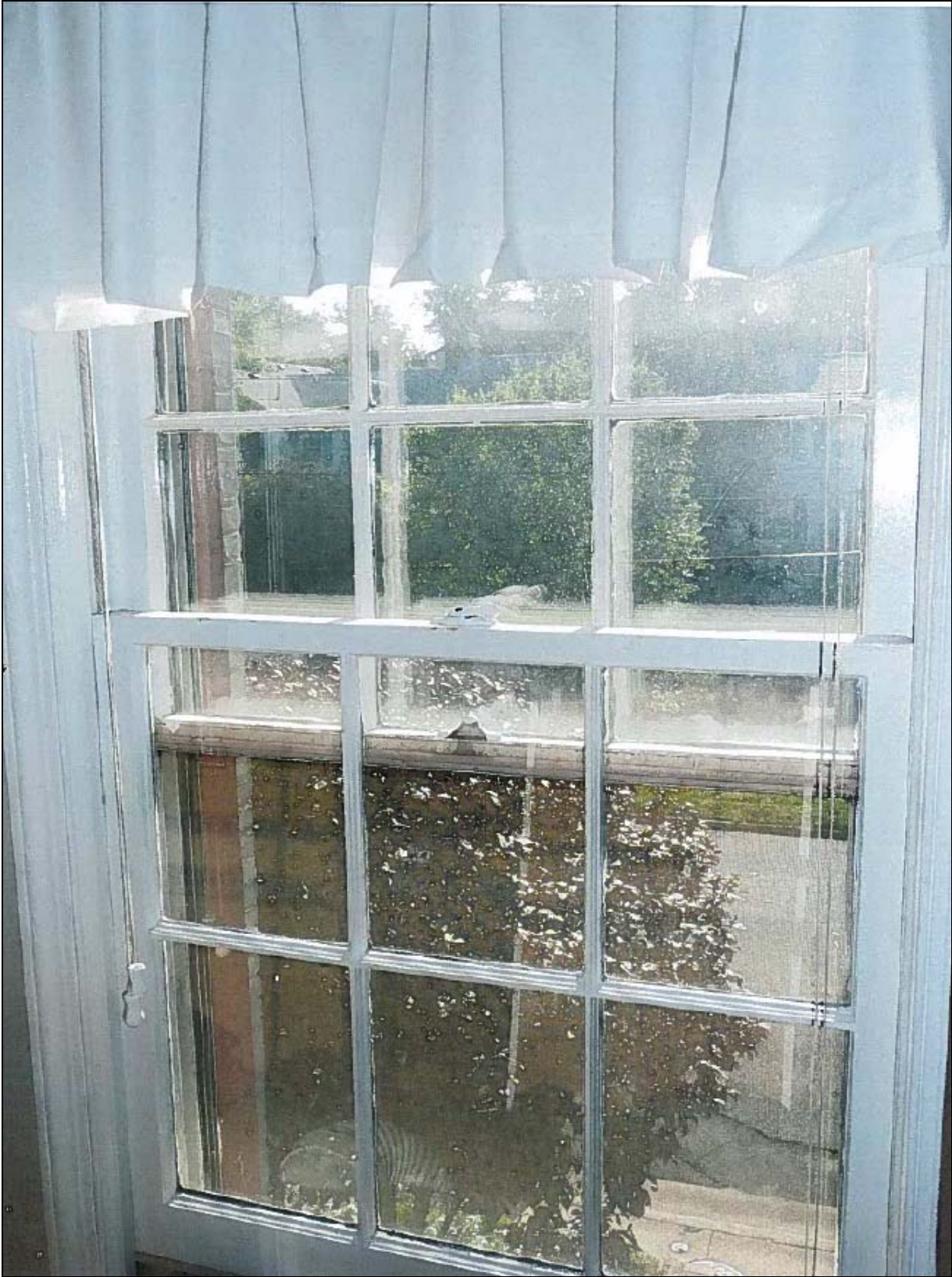
Figure 4. Interior view of window proposed for replacement on second story.
