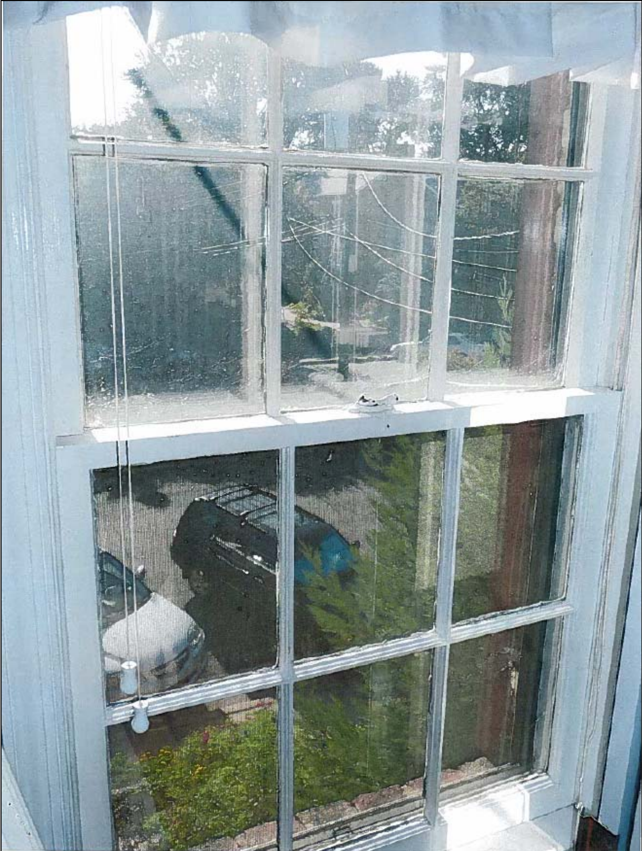
Figure 5. Interior view of window proposed for replacement on second story.
