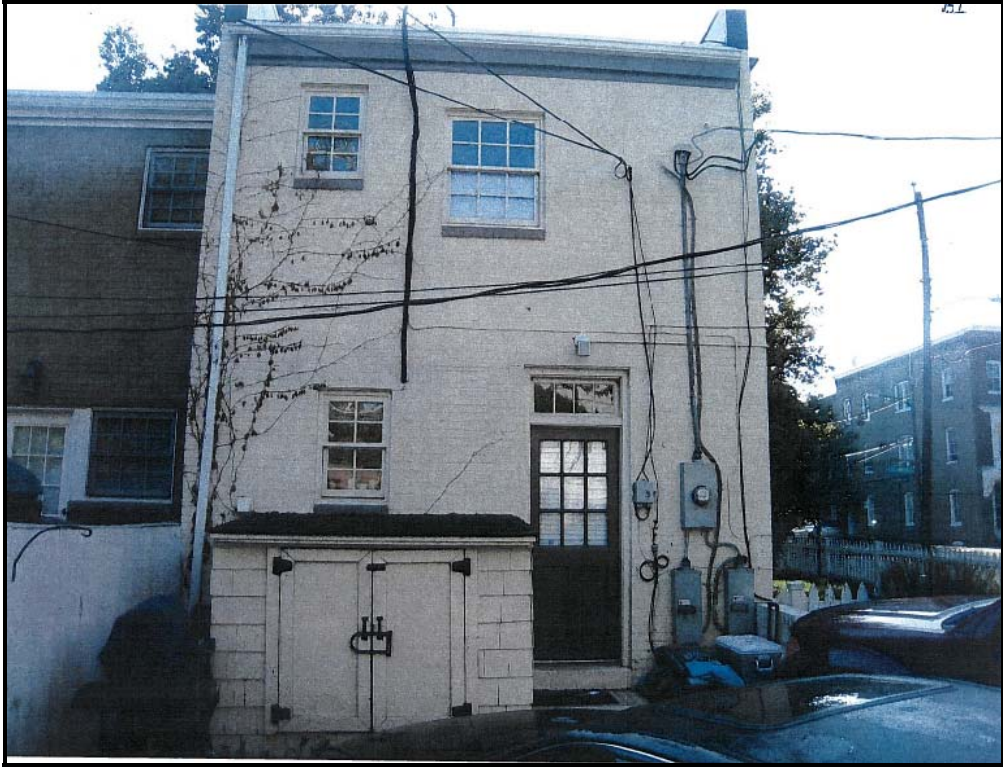
Figure 8: Existing Conditions - Rear Elevation
