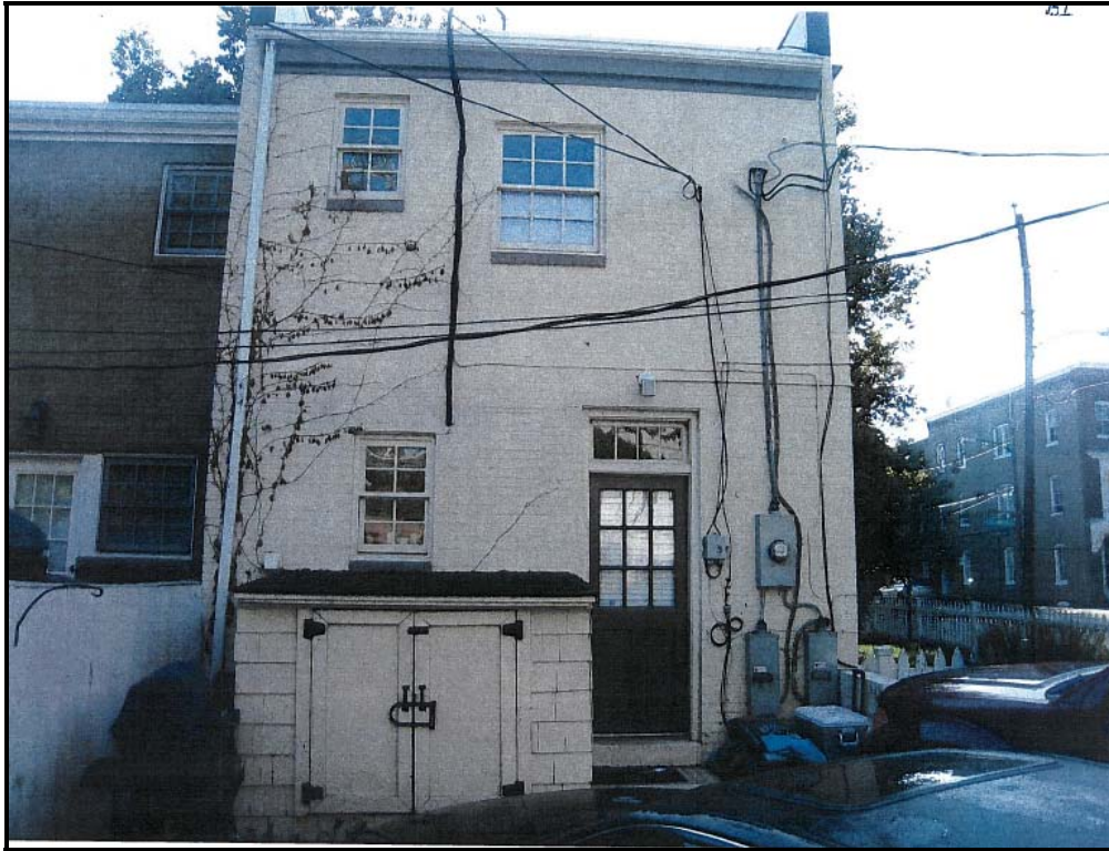
Figure 8: Existing Conditions - Rear Elevation
