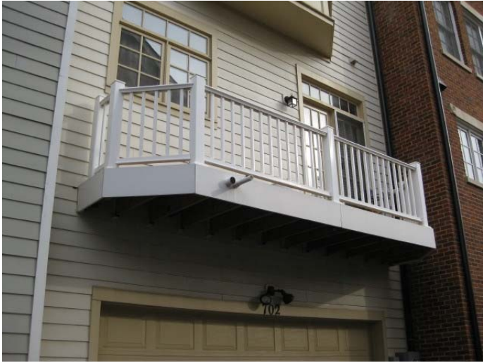
Figure 5: Photo of an existing deck in Potomac Greens.
