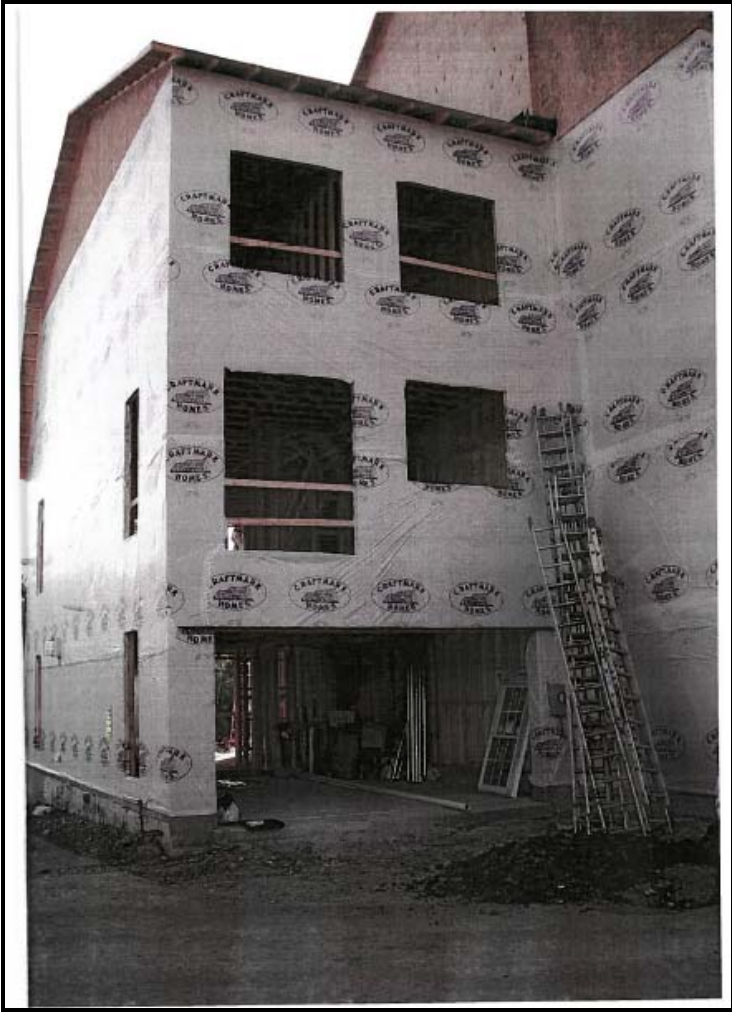
Figure 4: Photo of 1860 Carpenter Road under construction.
