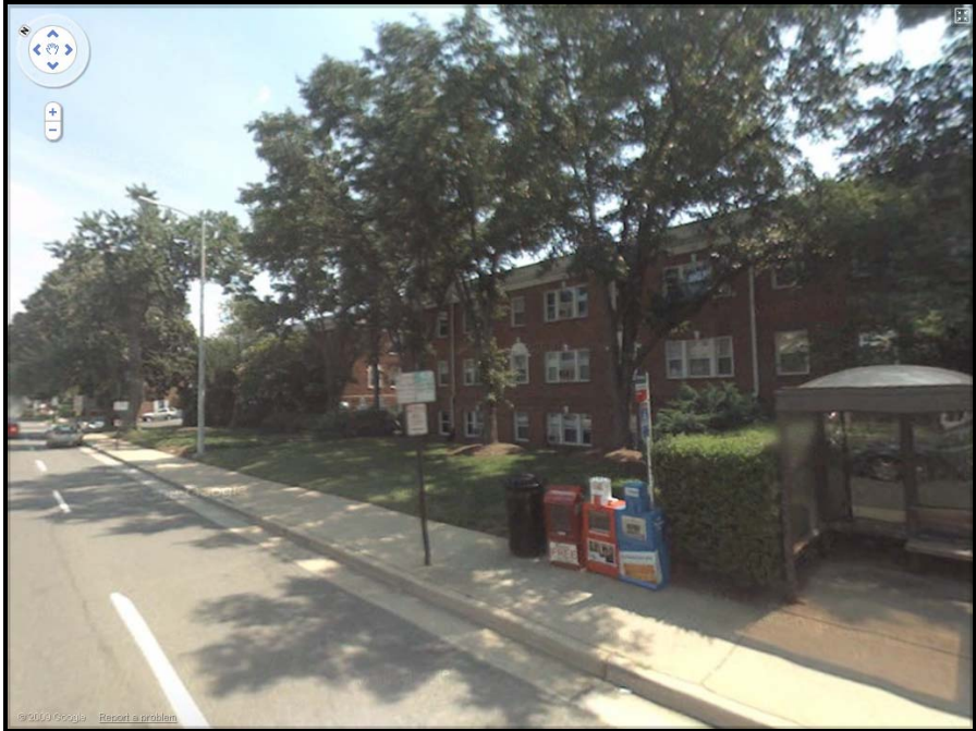
Figure 1. Photograph of building from S. Washington St.
