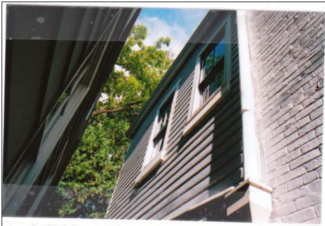
Figure 7. Windows on south elevation proposed for replacement.
