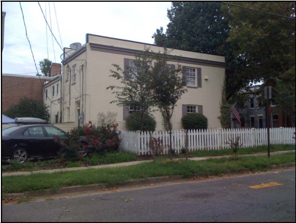
Figure 5: Existing Conditions – Side and Rear Elevations from Oronoco Street
