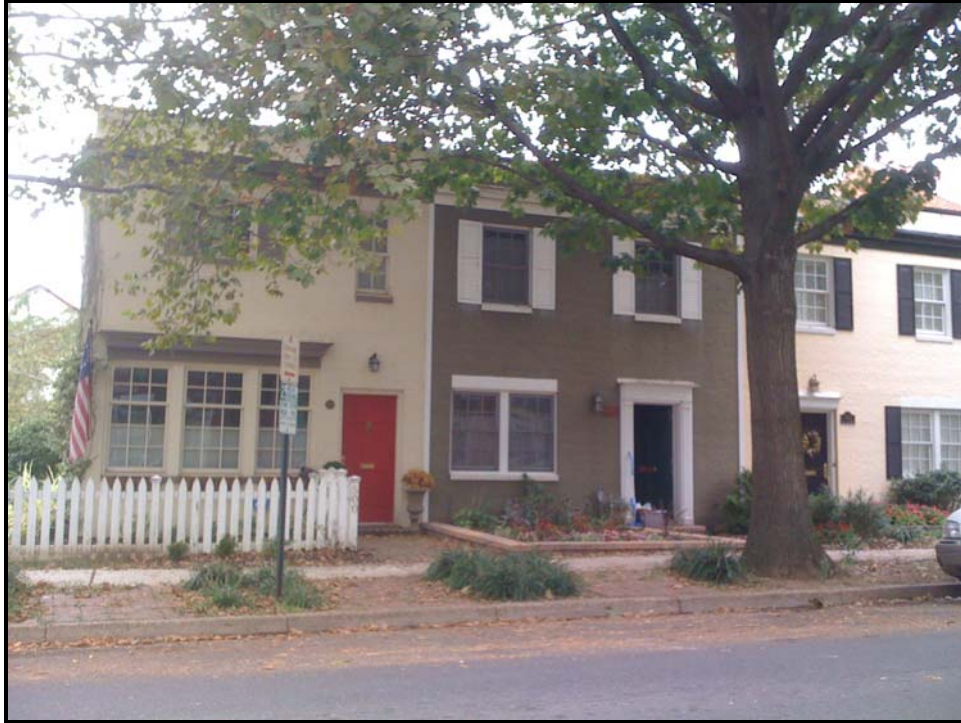
Figure 2: View of the three rowhouse sticks (c1963)
