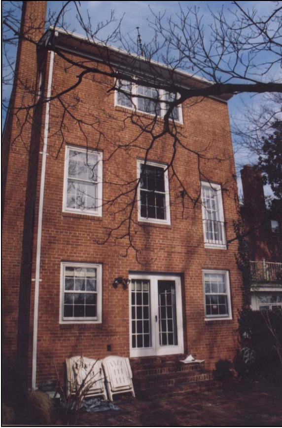
Figure 3. Existing south (rear) elevation.
