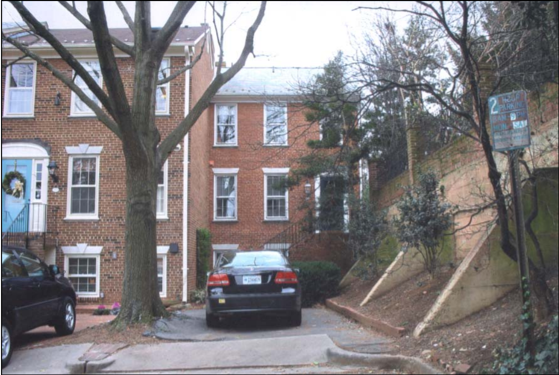
Figure 1. Existing north (front) elevation.
