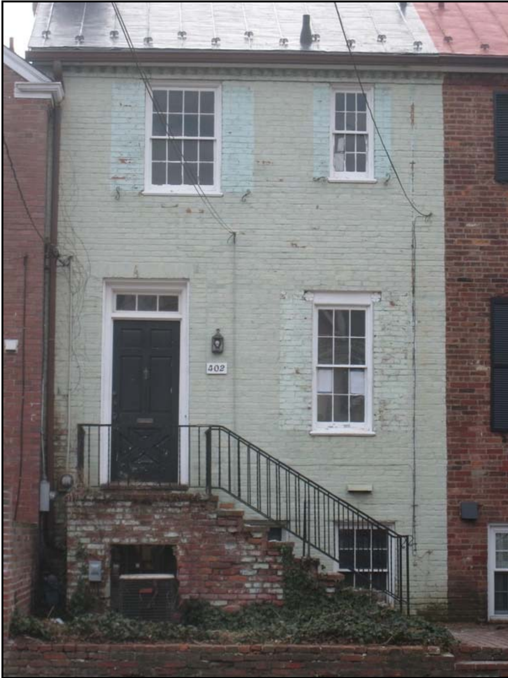
Figure 1. Front (north) elevation, 402 Jefferson Street, showing opening in stoop.
