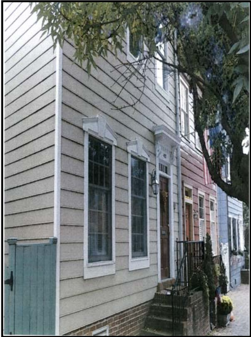
Figure 1: Photograph of front facade.
