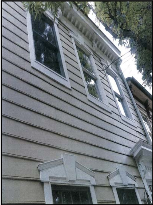
Figure 2: Detail of front facade.
