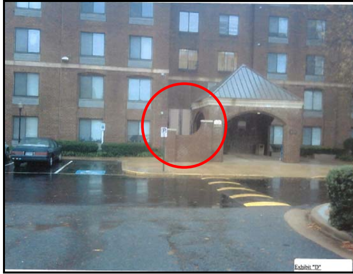
Figure 5: Existing Conditions - Front Elevation
