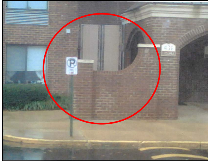
Figure 8: Existing Conditions - Front Elevation
