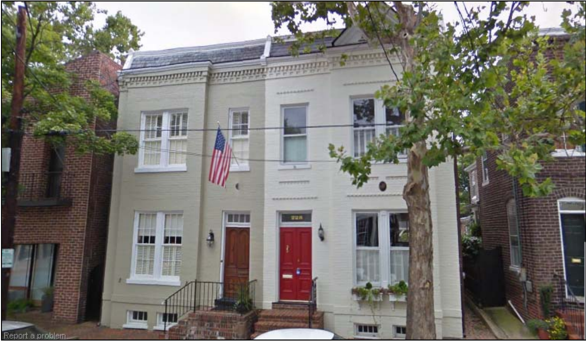
Figure 2: Existing Front Facade
