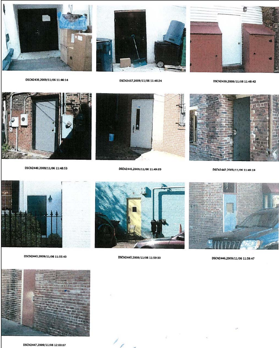
Figure 3. Photograph's submitted by applicant showing additional examples of flush metal doors on commercial buildings on Washington Street and King Street.
