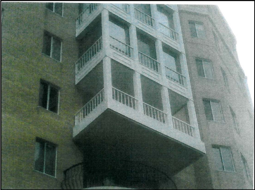
Figure 2: Photograph of balcony to be enclosed.
