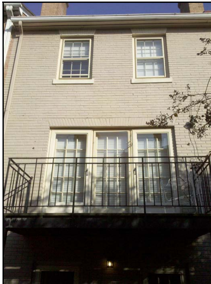
Figure 2: Photo of second and third floor rear elevation.
