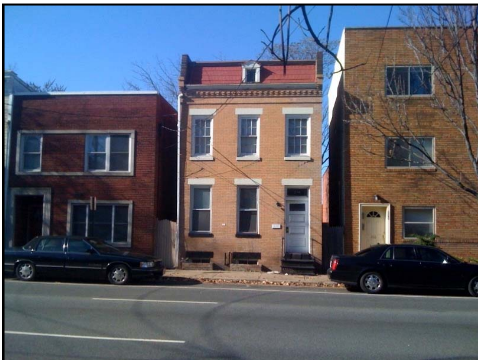
Figure 10: Photo of buildings across North Patrick Street.
