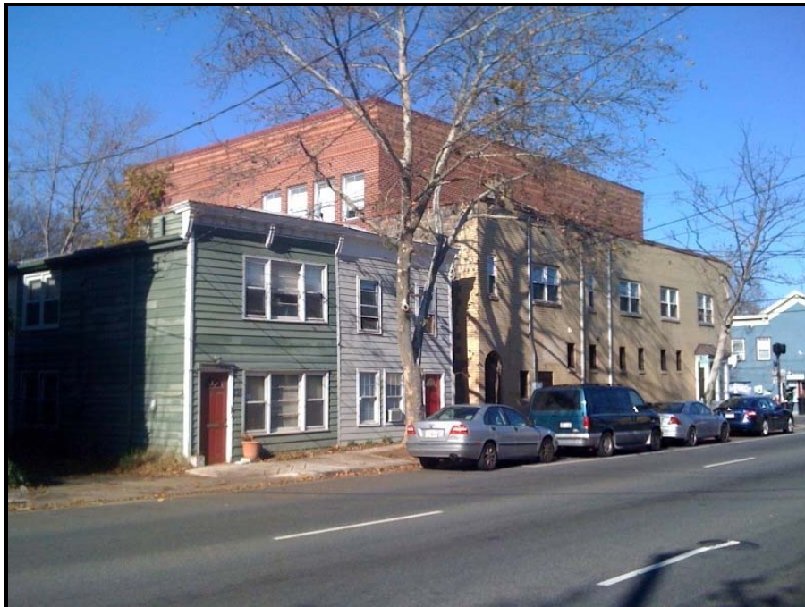
Figure 8: Photo of buildings across North Patrick Street.
