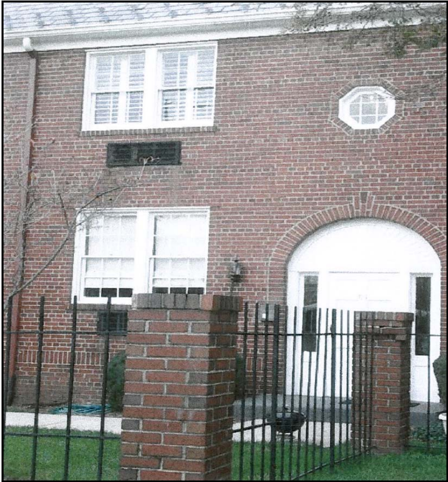
Figure 7: Front of Building – Windows after Aluminum Cladding
