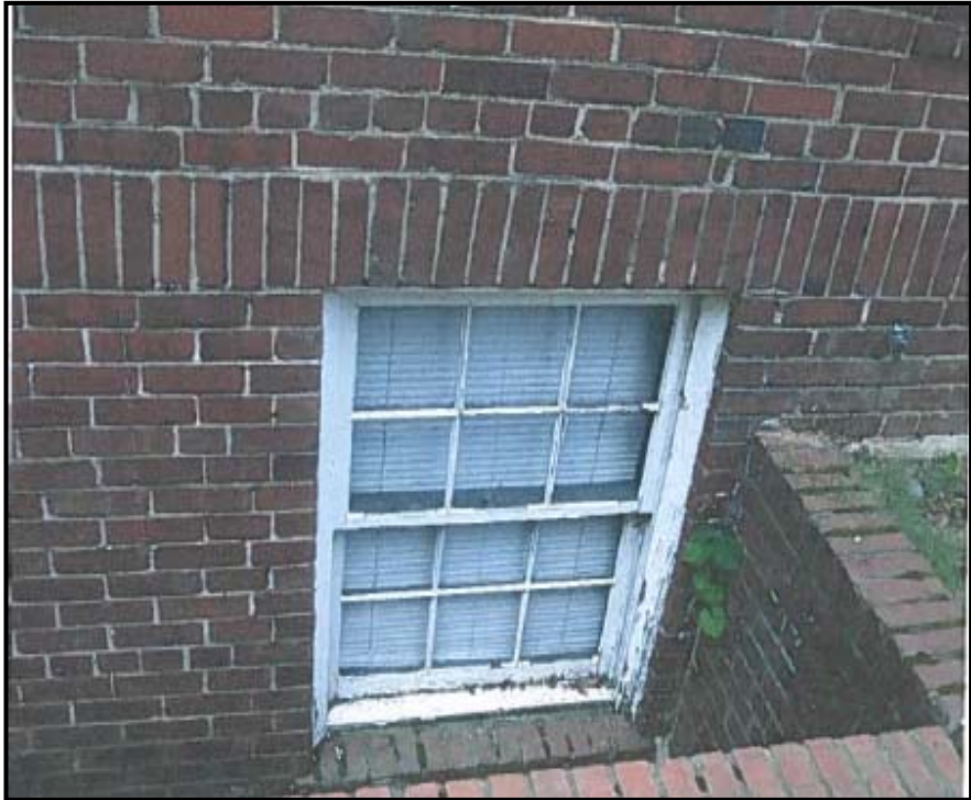
Figure 3: Before Aluminum Cladding
