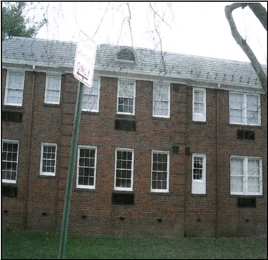
Figure 4: Rear of Building from a Distance
