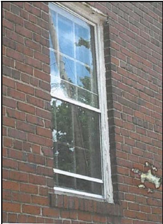
Figure 1: Before Aluminum Cladding
