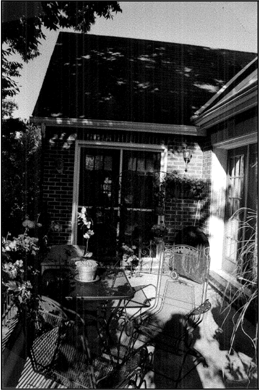
Figure 3. Portion of porch to be enclosed
