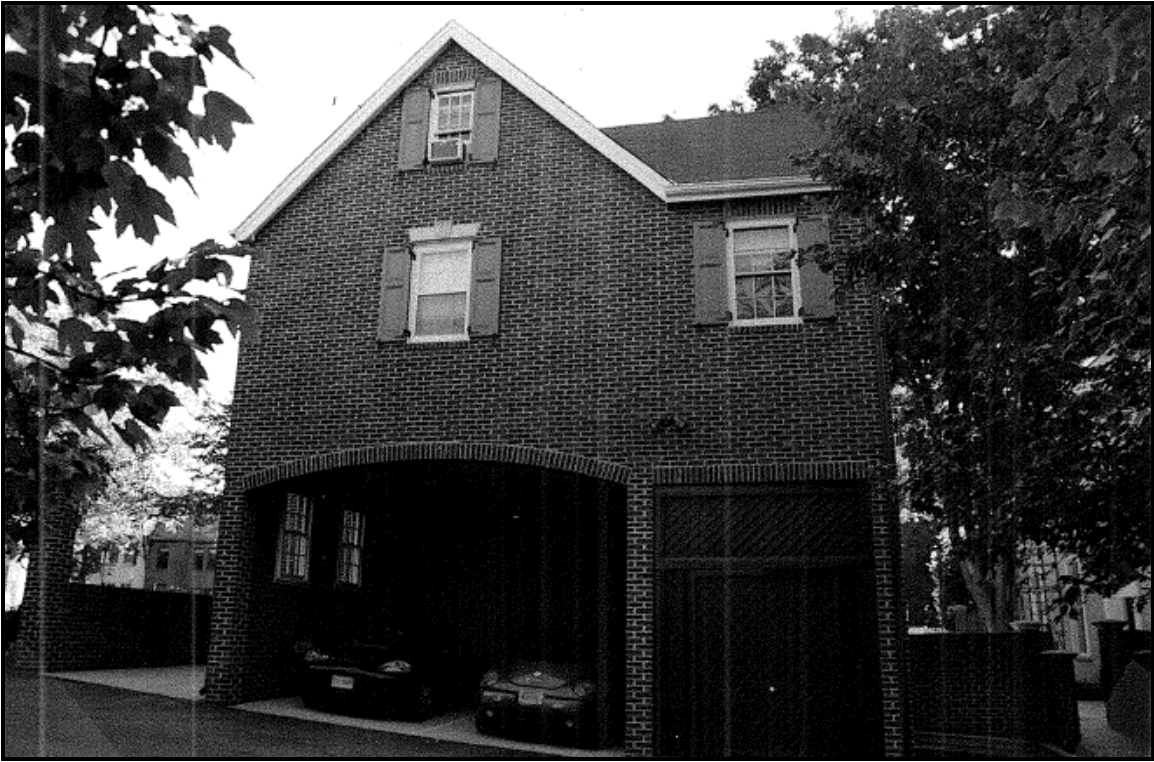
Figure 2. Image of west elevation
