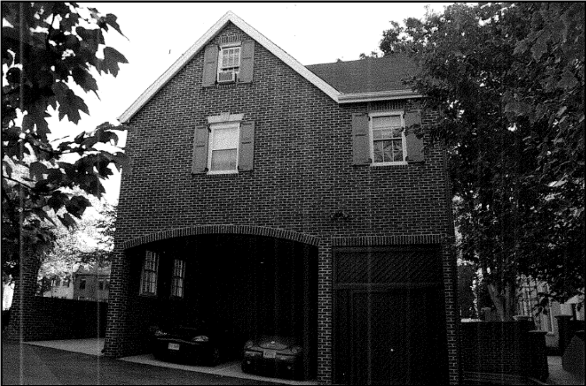
Figure 2. Image of west elevation
