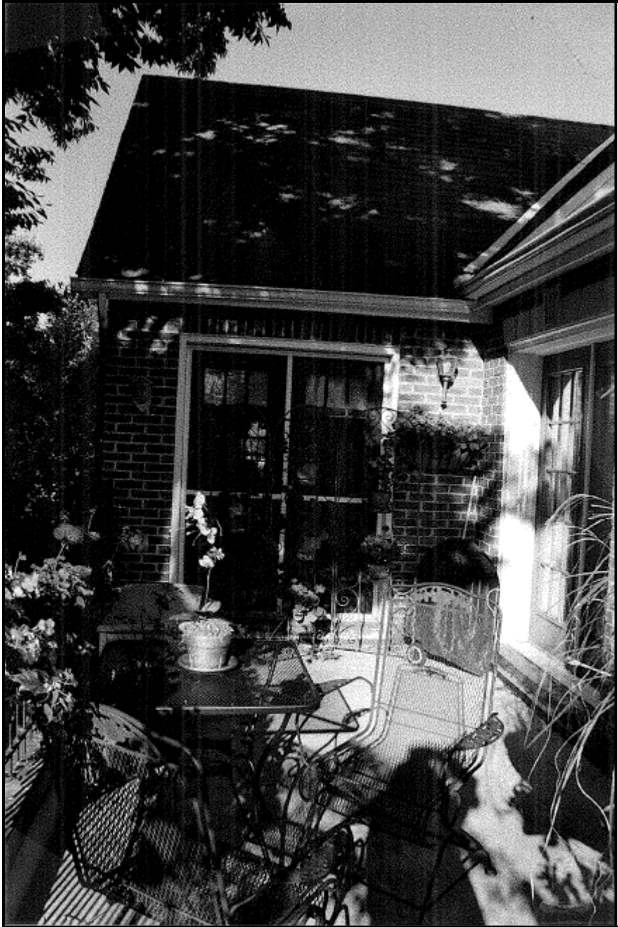
Figure 3. Portion of porch to be enclosed
