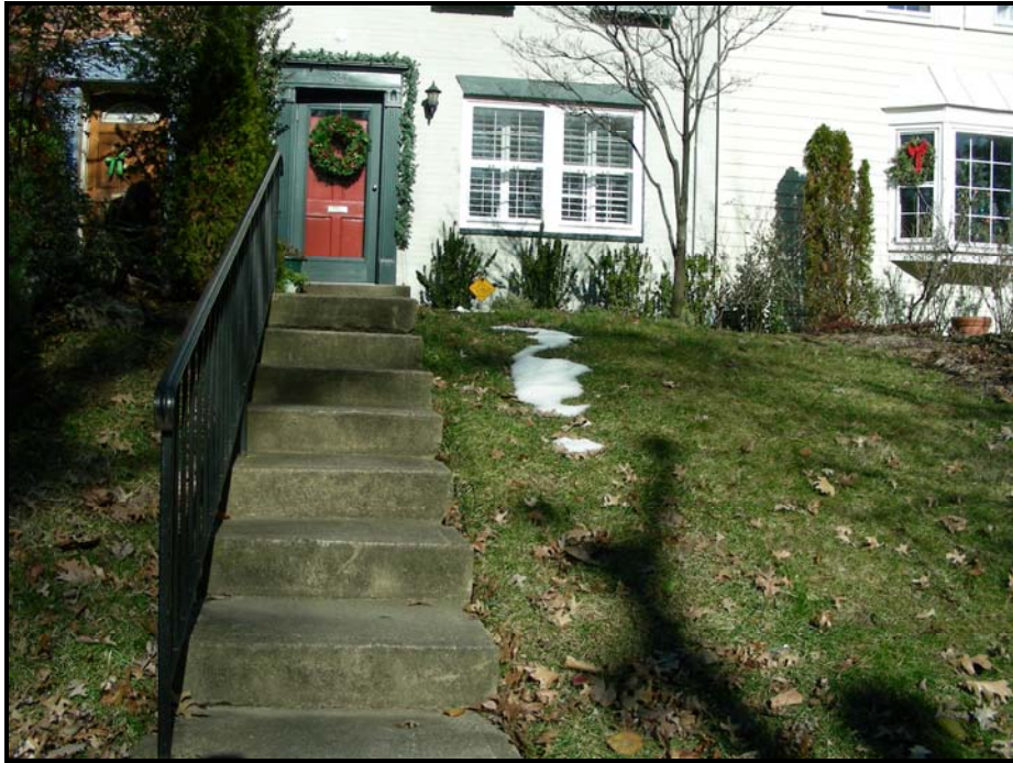
Figure 4: Photograph of existing stairs.
