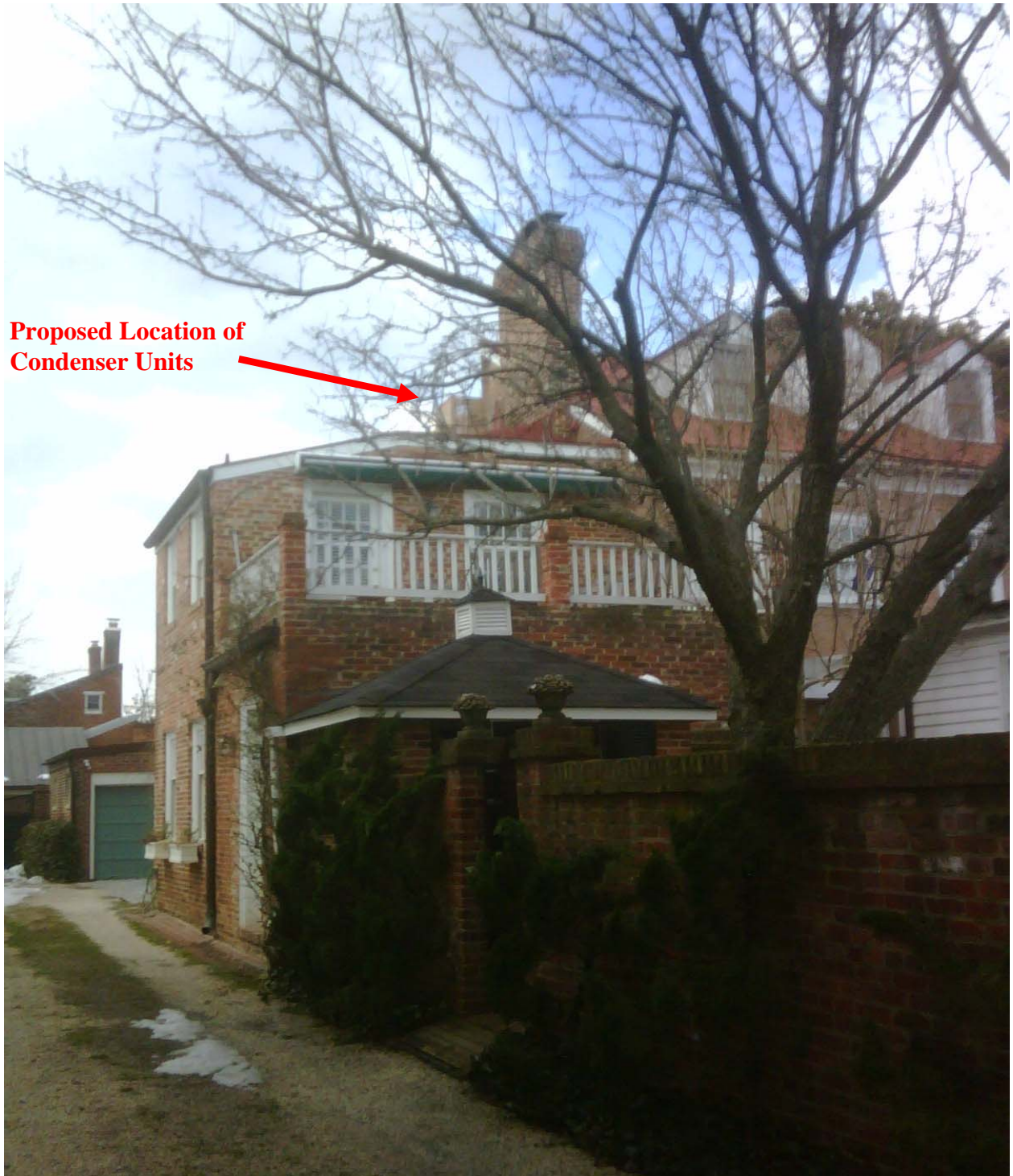
Figure 1: View of rooftop condenser mock-up from Lee St. looking west through the private alley
