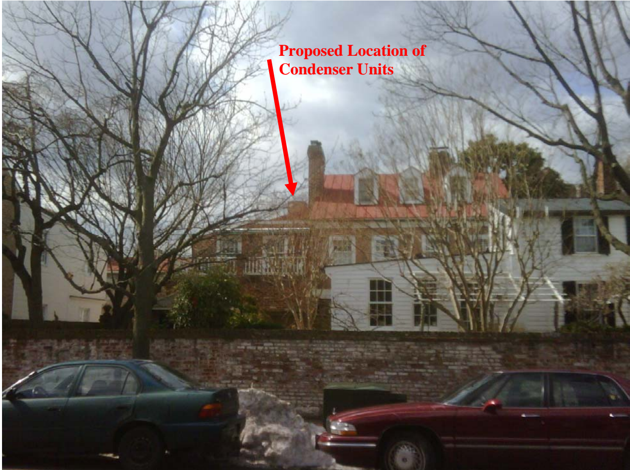
Figure 2: View of rooftop condenser mock-up from Lee Street ROW looking west
