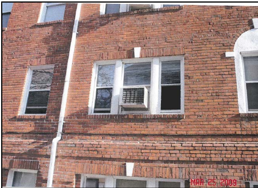
Figure 2. Photograph of building with existing HVAC units.
