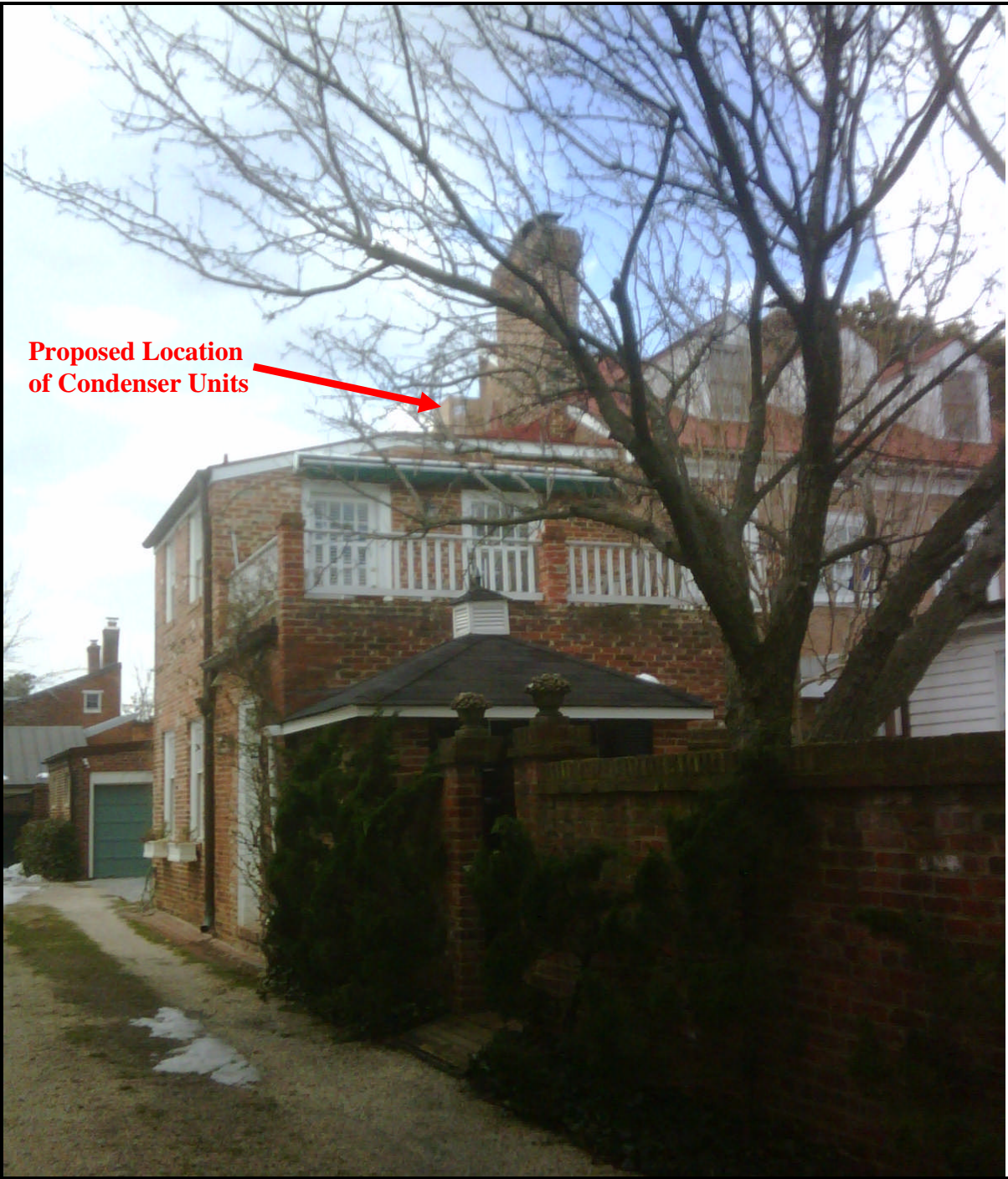
Figure 1: View of rooftop condenser mock-up from Lee St. looking west through the private alley
