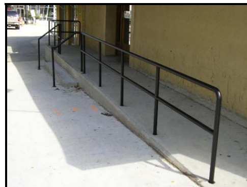
Photo of an open metal handrail
