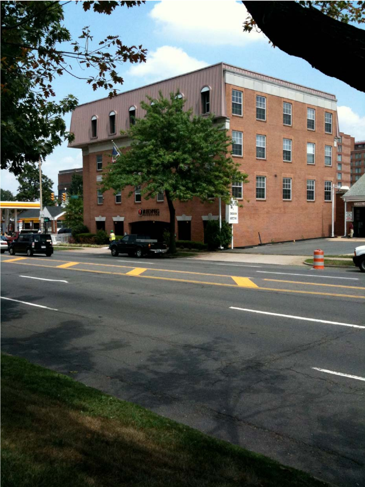
Figure 1. Existing signage on N. Washington elevation.
