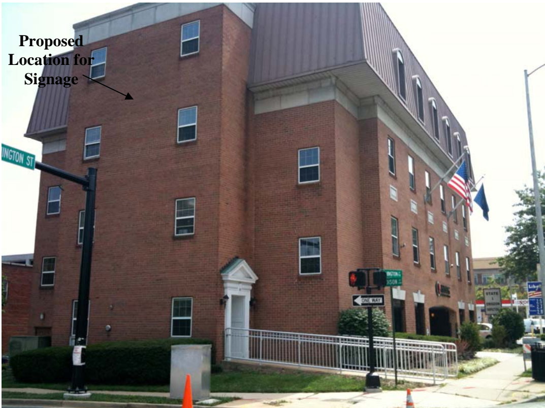
Figure 3. Madison Street elevation showing proposed signage location and unapproved balustrade
