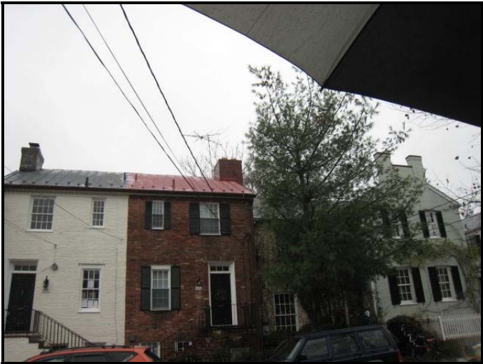
Figure 2. Front facade of 404 Jefferson St.
