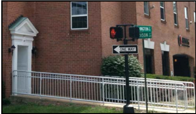
Photo of existing white metal balustrade
