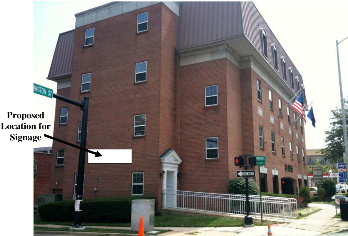
Figure 3. Madison Street elevation showing proposed signage location and unapproved balustrade
