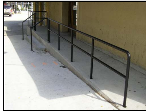
Photo of an open metal handrail
