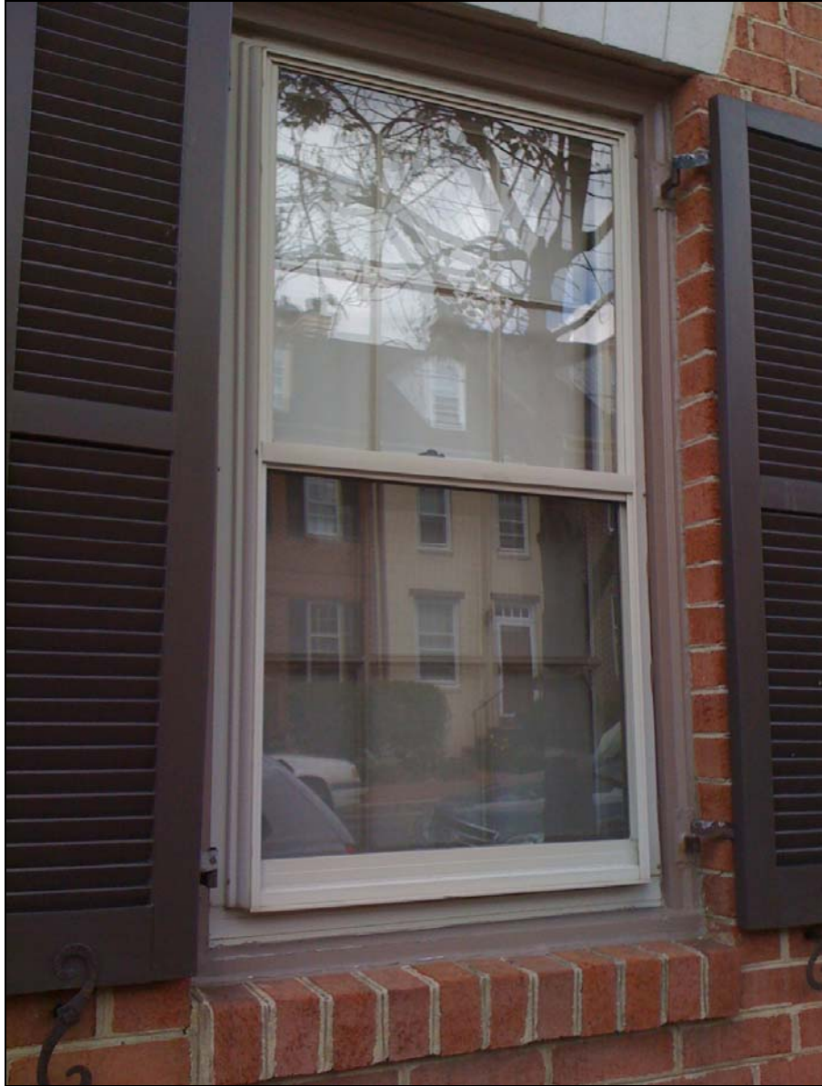
Figure 3: Example of Existing Single Glazed Windows with Storms
