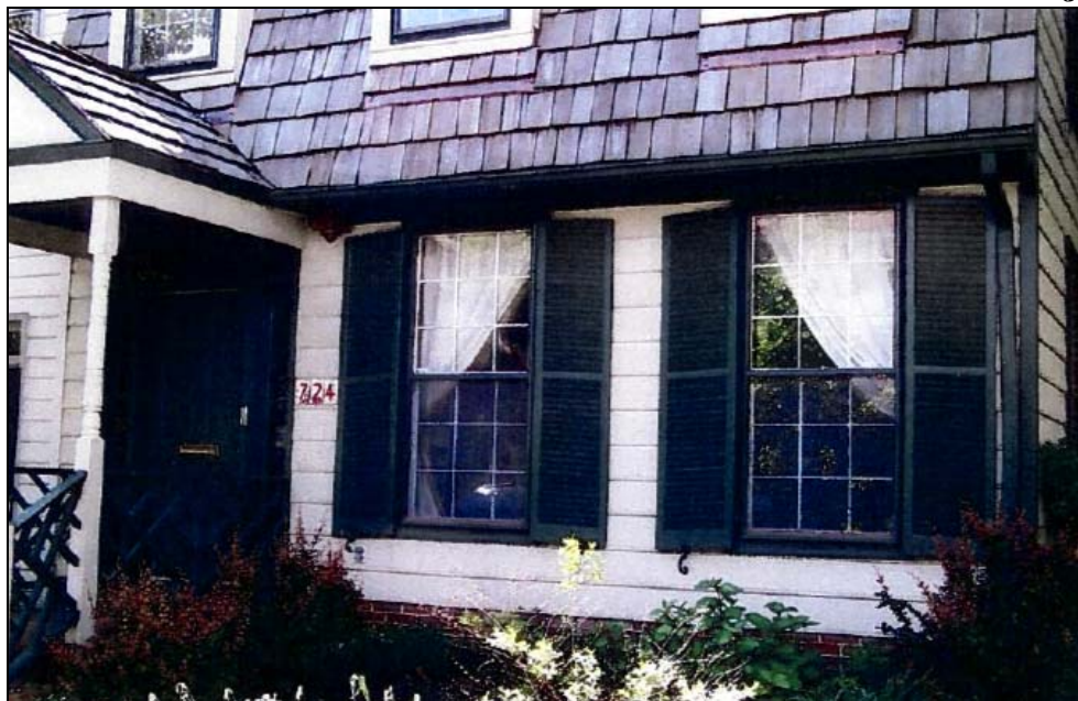
Figure 3: Photograph of Existing Windows
