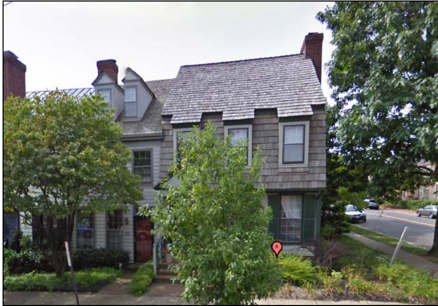
Figure 1: Photograph of Existing Windows – Front Elevation/Gibbon St.
