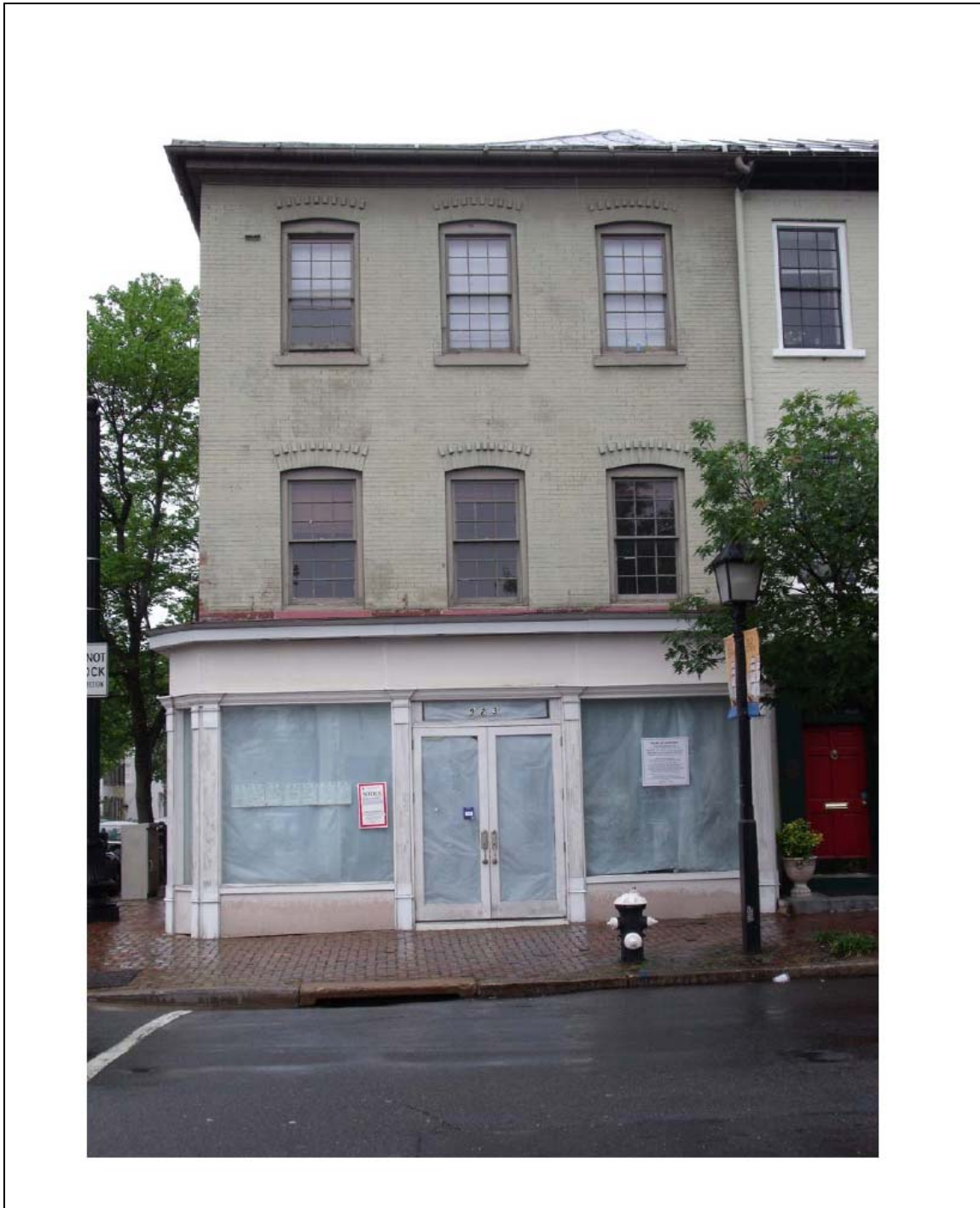
Figure 6: Existing Photo - Front Elevation
