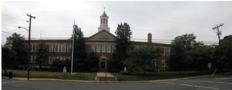
St. Mary's main building Green Street elevation.
