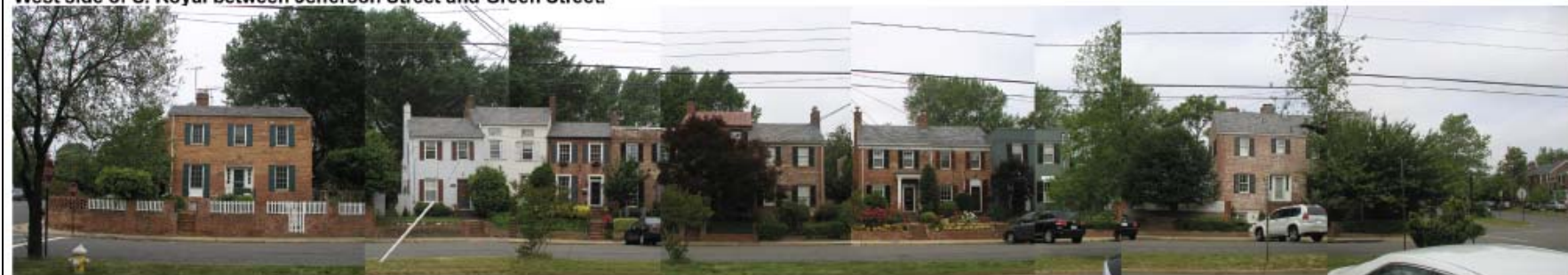
North side of Green Street between S. Pitt Street and S. Royal Street.
