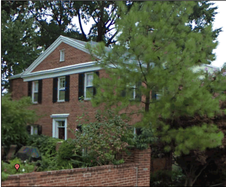
Figure 1: Photograph of Existing Windows – Front Elevation/Green Street
