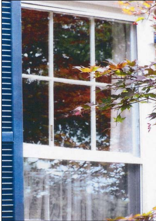
Figure 3: Photograph of Existing Windows
