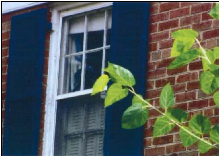
Figure 4: Photograph of Existing Windows
